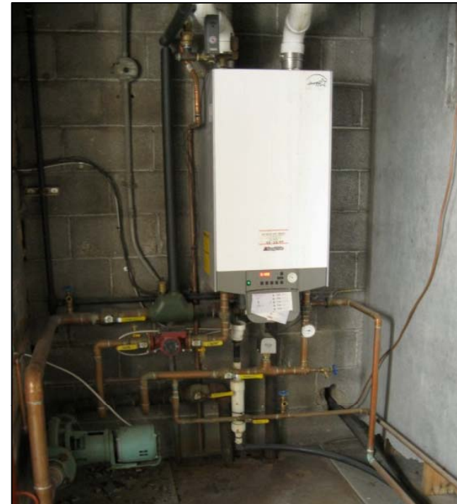
High Efficiency Hot Water Boiler
